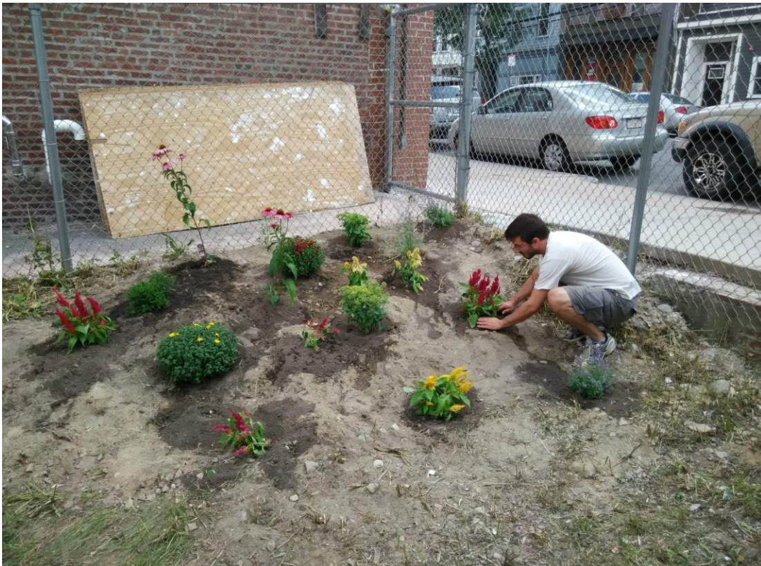
FIGURE A RAIN GARDEN -- FED BY RAIN WATER RUNOFF FROM THE STREET
